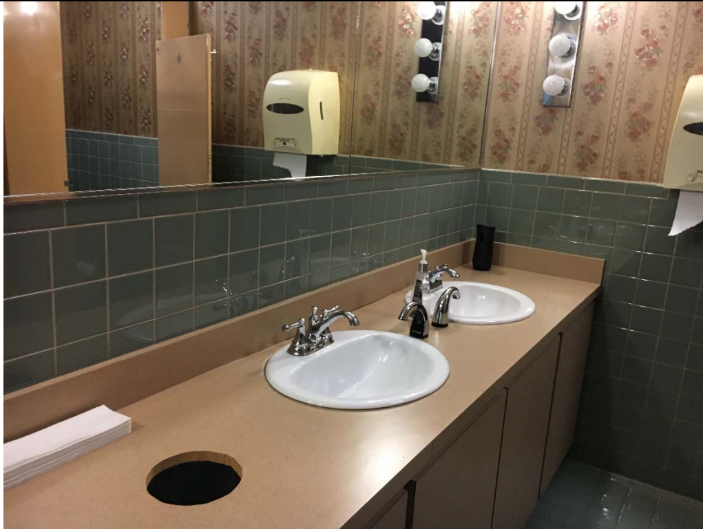
Violation 27 - Second Floor Women's room - Lavatory does not have the required toe and knee clearance provided.
