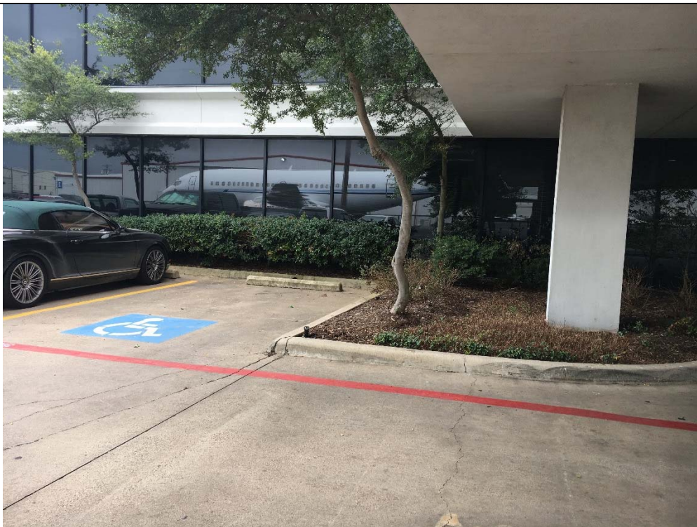
Violation 2 - Only one accessible parking space is provided where two are required and one of the two is required to be van accessible.
