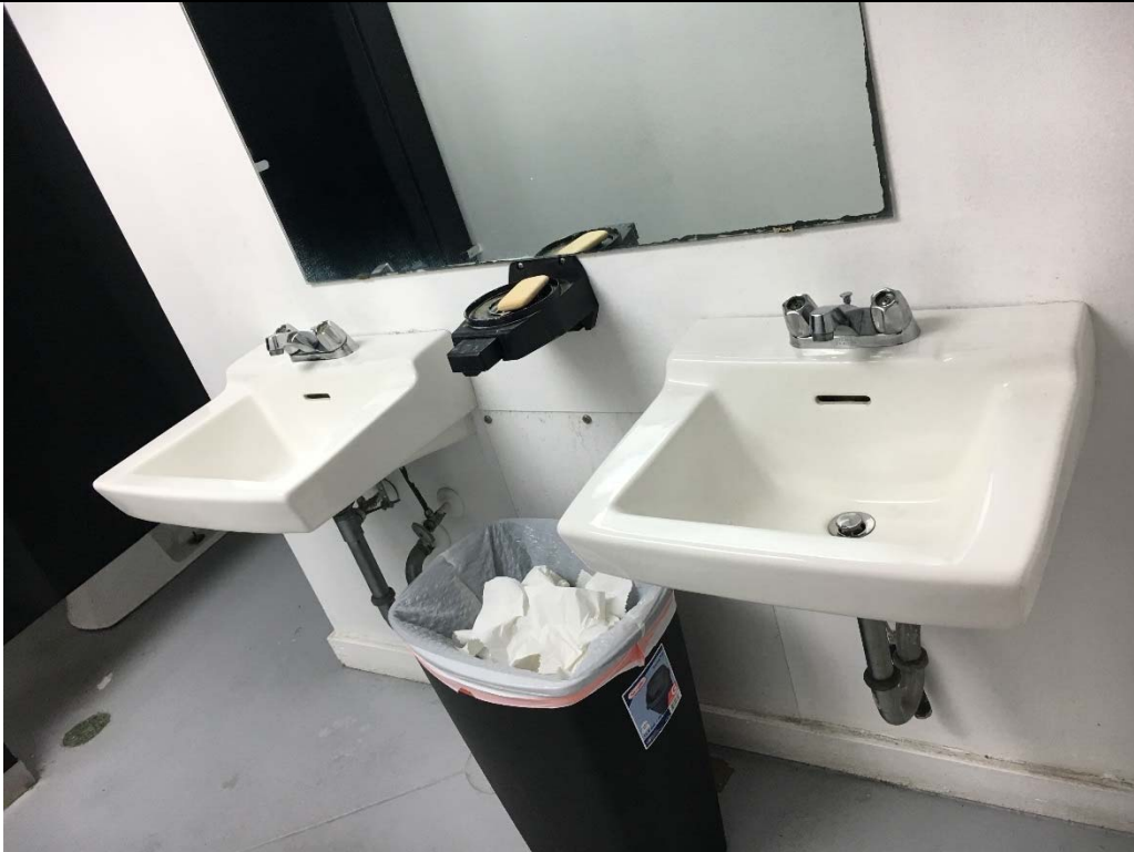
Violation 30 - The warehouse restroom does not have an accessible lavatory provided.
