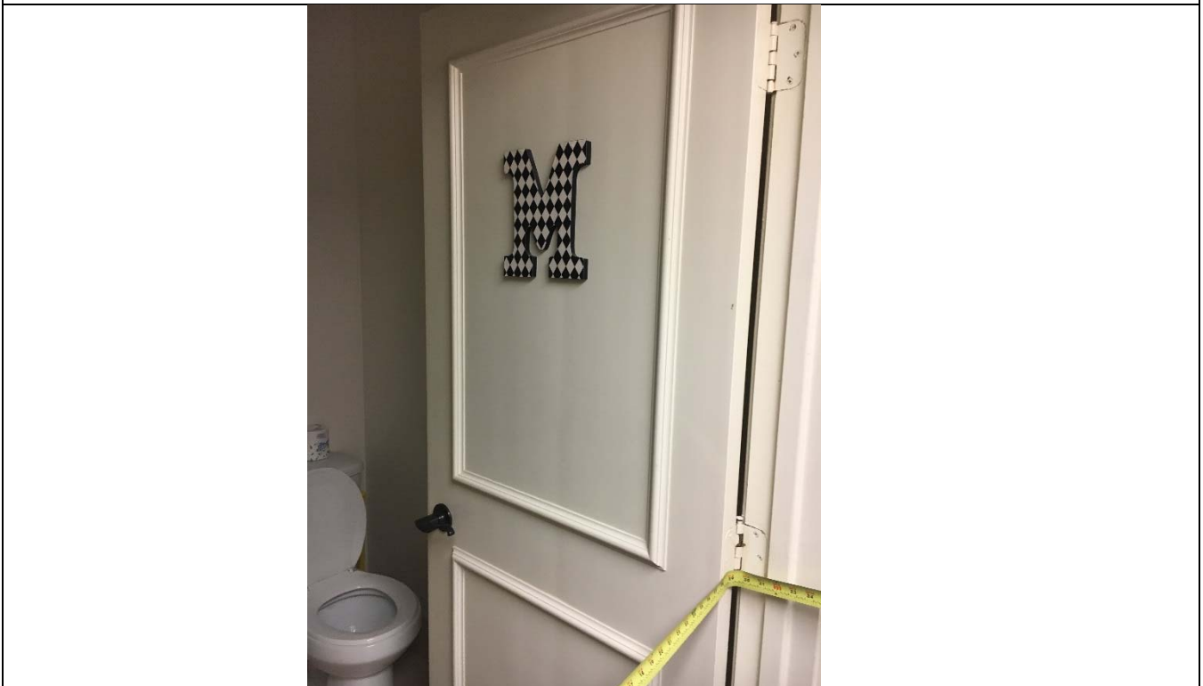
Violation 14 - The Women's restroom on the first floor is too small and does not have the required turning radius provided.
