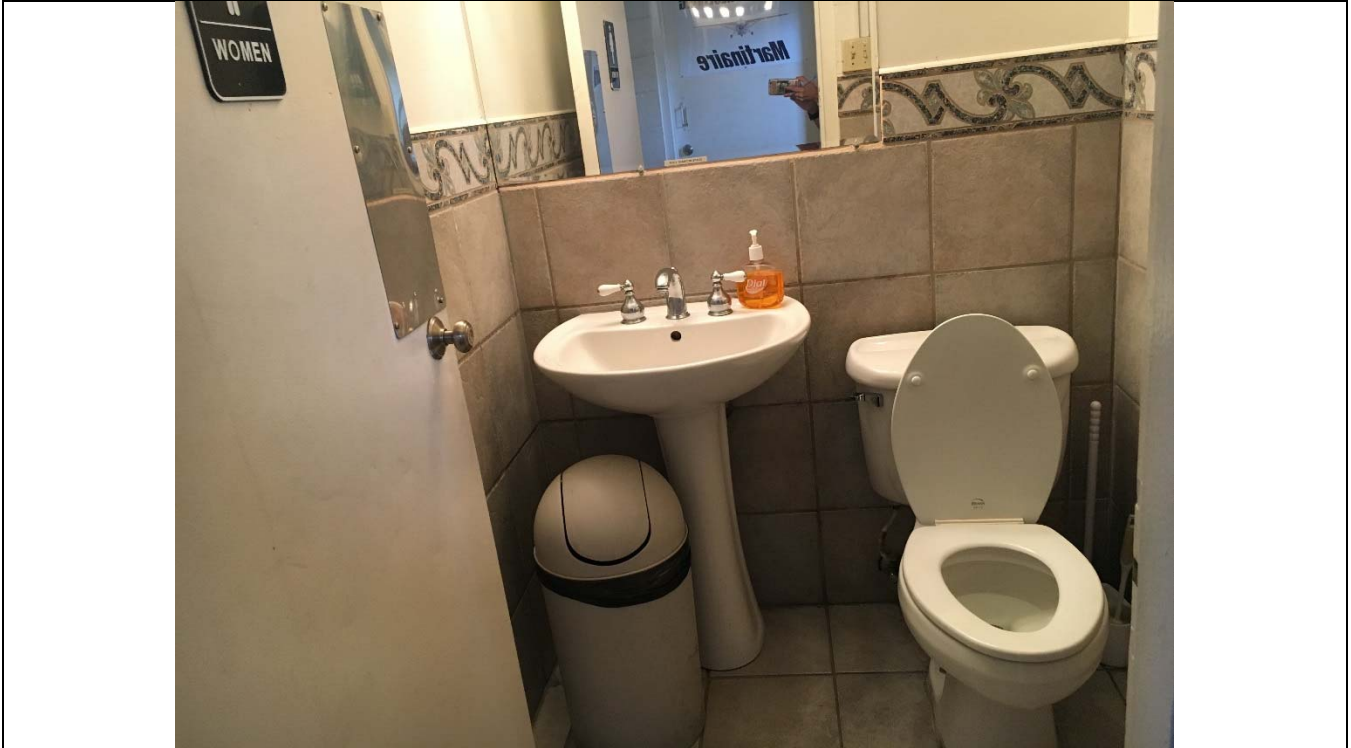
Violation 14 - The Women's restroom on the first floor is too small and does not have the required turning radius provided.
