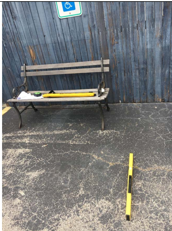
Violation 2 - The left accessible space has a 3.5% running slope.
