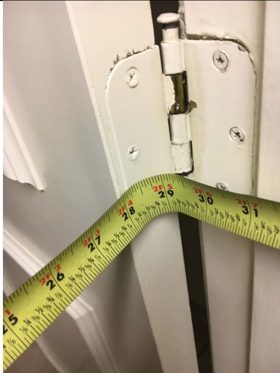
Violation 15 - Men's and Women's restroom doors on the 2nd floor only have a 28" opening.
