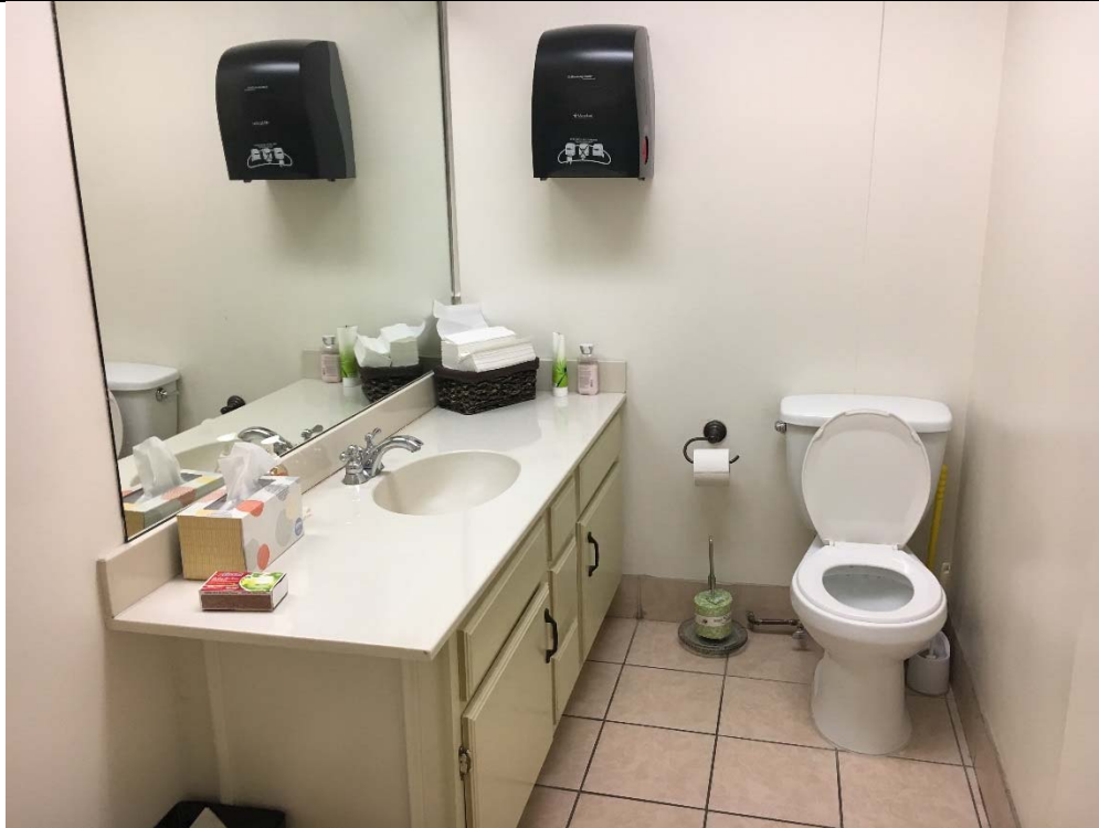
Violation 17 - The Women's restroom on the second floor is too small and does not have the required turning radius provided.
