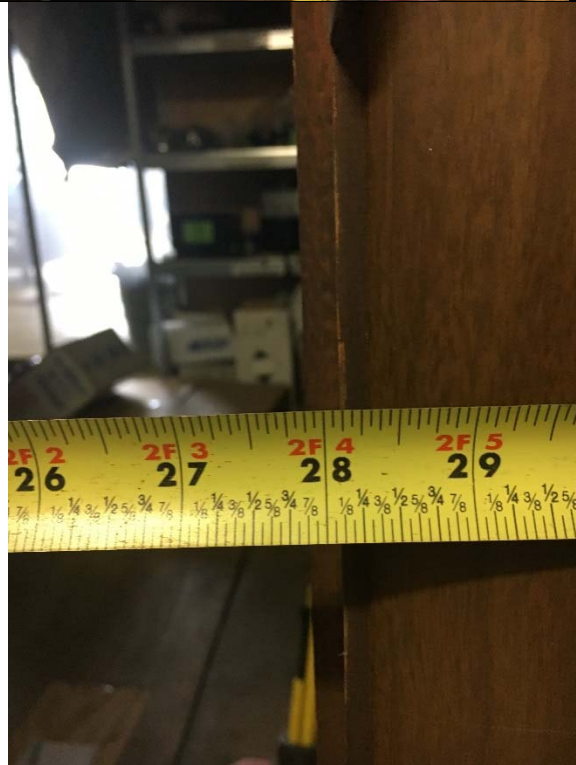
Violation 12 - The entrance into the storage room has an opening of only 28" wide.
