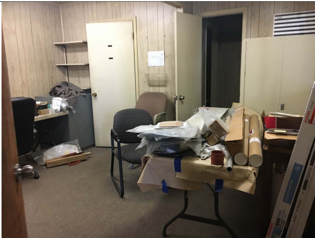
Violation 6 - The two interior doors have door hardware that requires grasping and twisting to operate.
