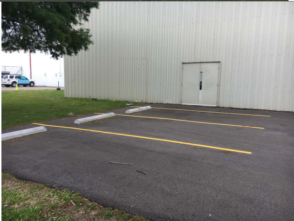
Violation 1 – Eight parking spaces serve this building and none are accessible.
