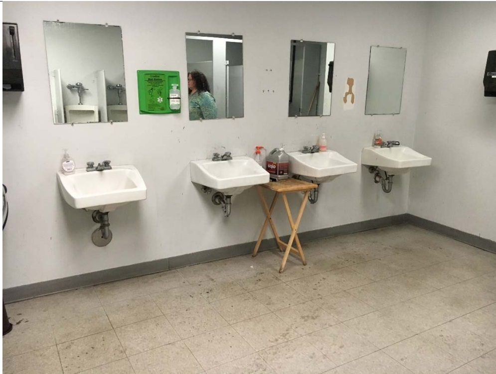
Violation 5 - Men's Restroom: There are 4 lavatories provided and none of them have any compliant features.
