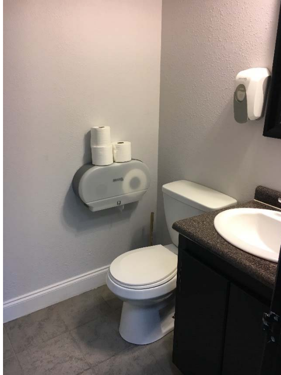
Violation 10 - The Women's single user restrooms is not large enough to accommodate a wheelchair turning space.
