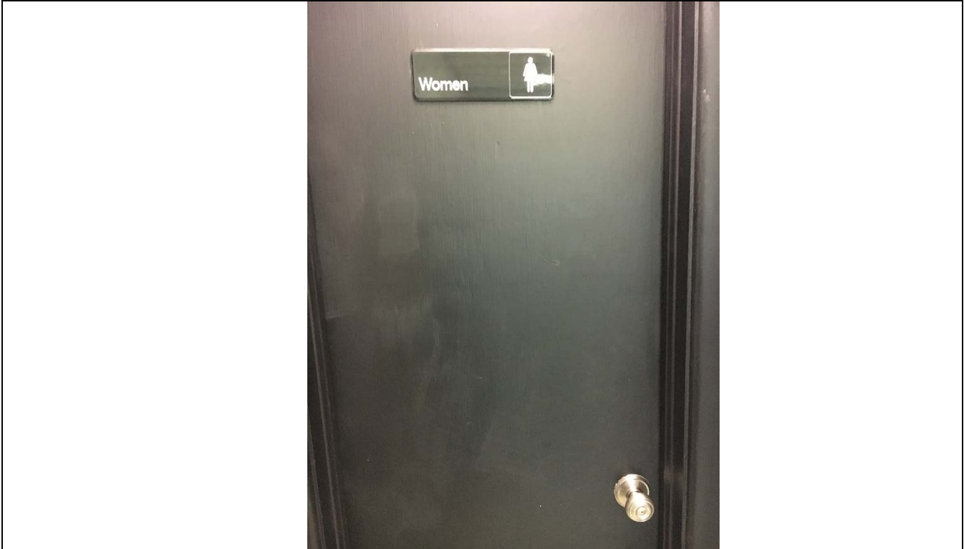
Violation 8 - Men's and Women's Restrooms: Door hardware requires grasping and twisting to operate.
