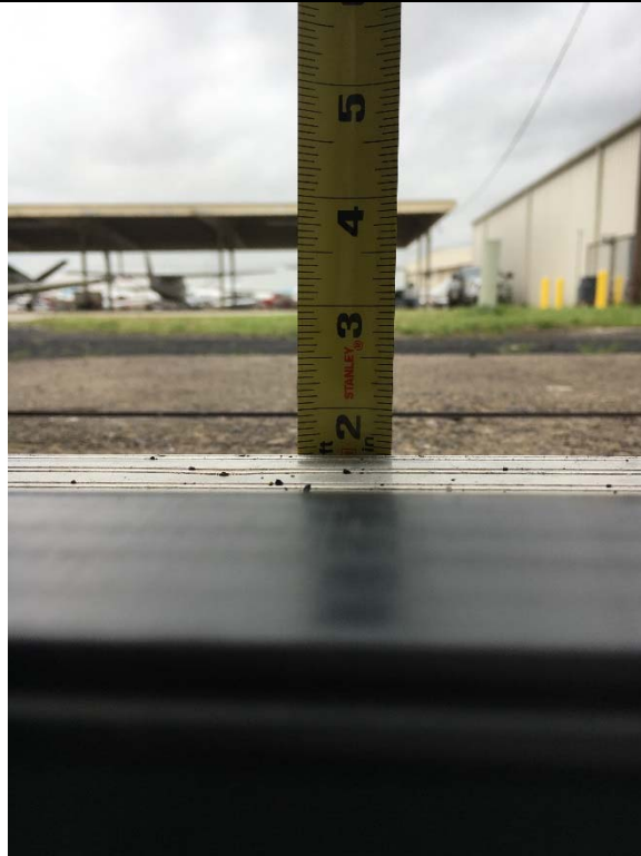
Violation 6 - The route leading outside from the Testing Center has a 1-1/2" step down.
