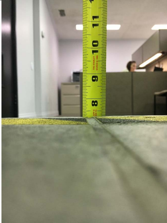
Violation 5 - The route leading into the Testing Center requires a 7-5/16" step down to enter.
