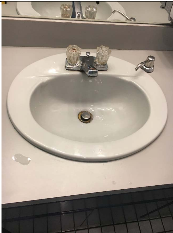
Violation 16 - Men's Room: The lavatory faucets controls require grasping and twisting to operate.
