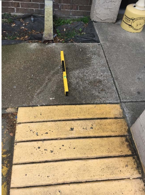
Violation 5 - The sidewalk as well as the landing at the top of the curb ramp has a 5.4% cross slope.
