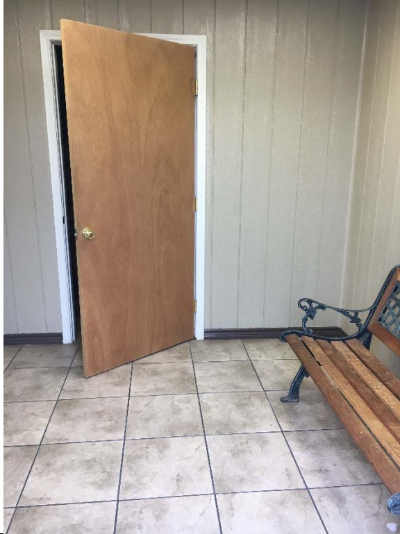
Violation 2 - The restroom door has door hardware that requires grasping and twisting to operate.
