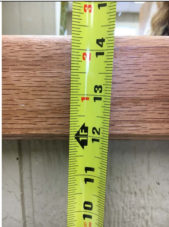
Violation 6 - The mirror is mounted at 49" to the bottom of the reflective surface.
