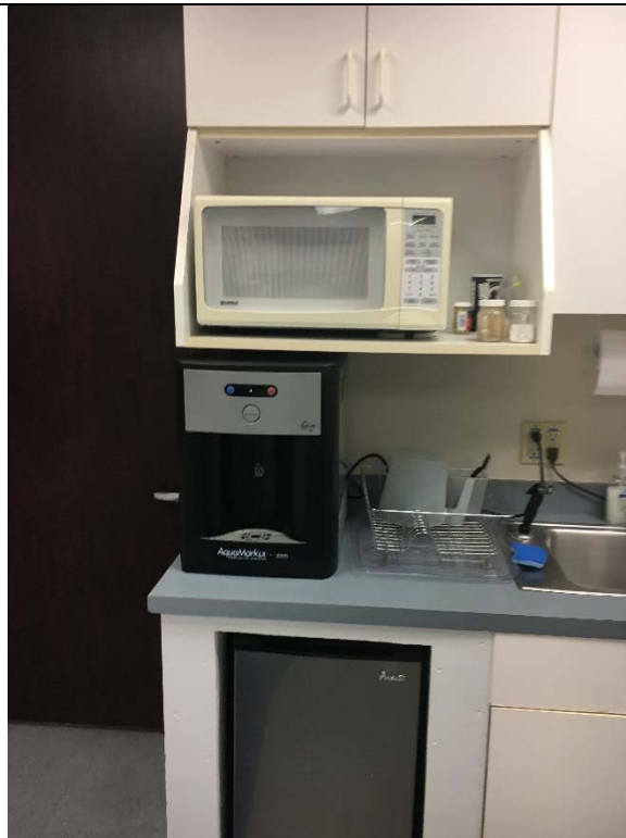
Violation 21 - The counters in the break room are from 35" to 36" above finished floor.
