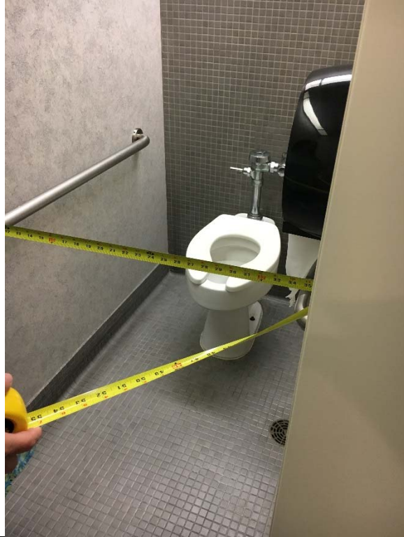
Violation 19 - Men's Restroom - No accessible stall provided; only an ambulatory stall is provided.
