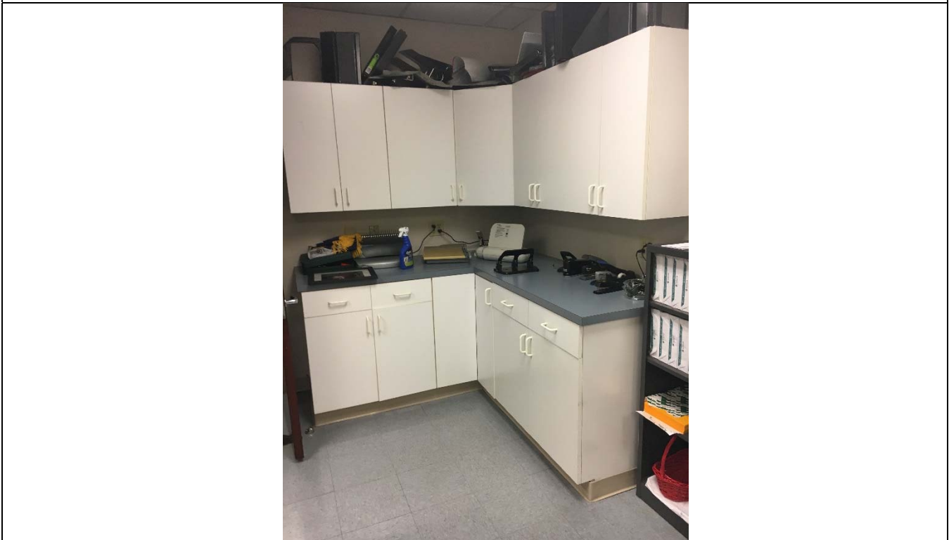
Violation 20 - The counter in the break room is 35-3/4" above finished floor to the top of the counter at the sink where a maximum of 34" is required.
