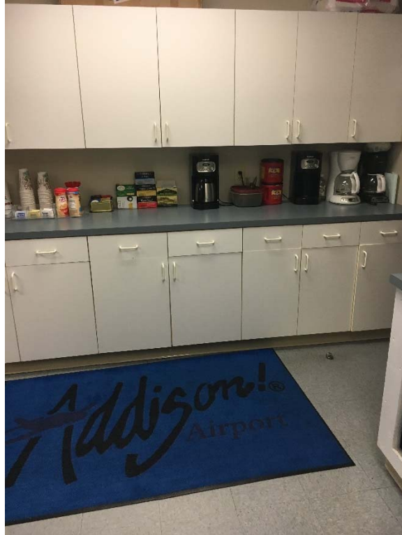
Violation 21 - The counters in the break room are from 35" to 36" above finished floor.
