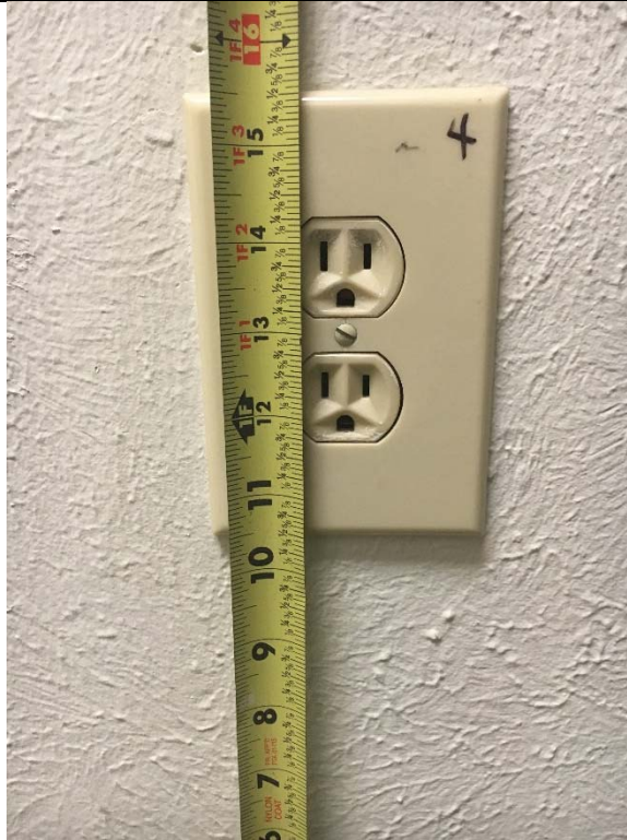
Violation 14 - Some outlets in the facility are mounted with the highest operable parts below the minimum requirement of 15" above finished floor.
