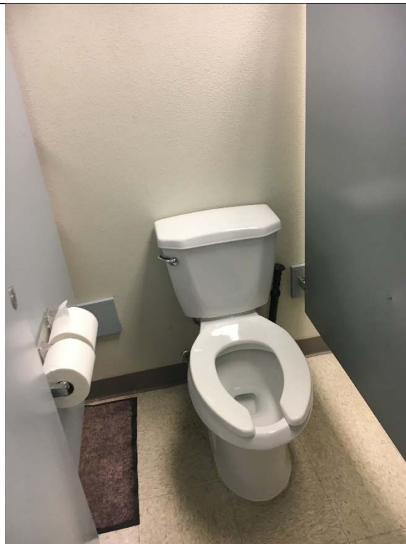
Violation 40 - Men's Restroom second floor of 4310 - Does not have an accessible stall provided.
