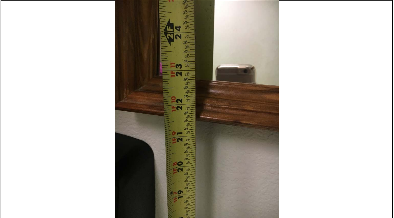
Violation 36 - Women's Restroom second floor of 4310 - The mirror is mounted at 52" above finished floor.
