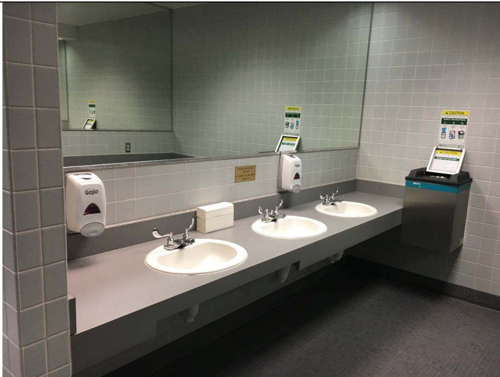
Violation 33 - Women's Locker Room - Mirrors are mounted higher than 40" to the bottom of the reflective surface.
