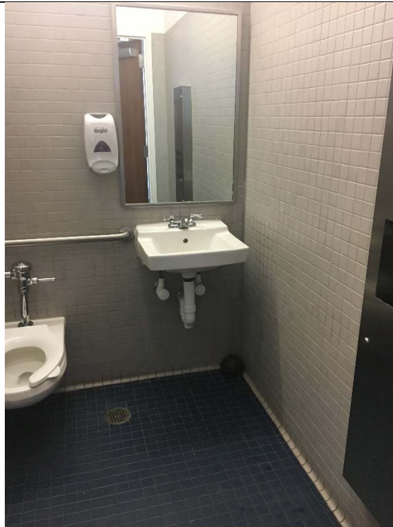
Violation 26 - 2nd floor Men's and Women's restrooms by the track - The lavatories encroach on the required clear floor width of the water closets.
