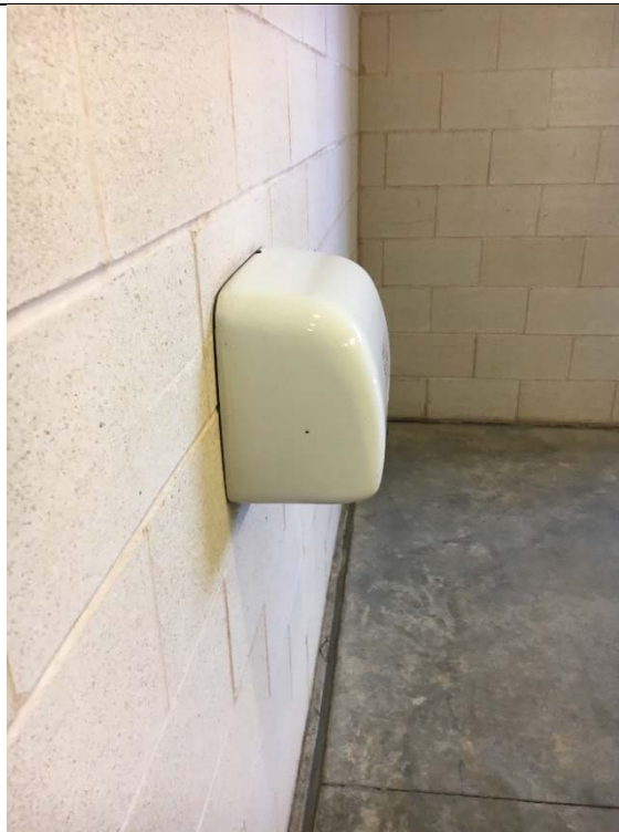
Violation 44 - Men's and Women's restrooms in pool area - Hand dryers protrude into the path of travel 7".
