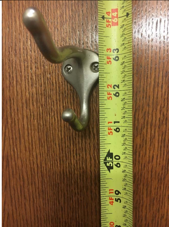
Violation 28 - 2nd floor Men's and Women's restrooms by track - Coat hooks are mounted with the highest operable part at 63" where a maximum of 48" is required.
