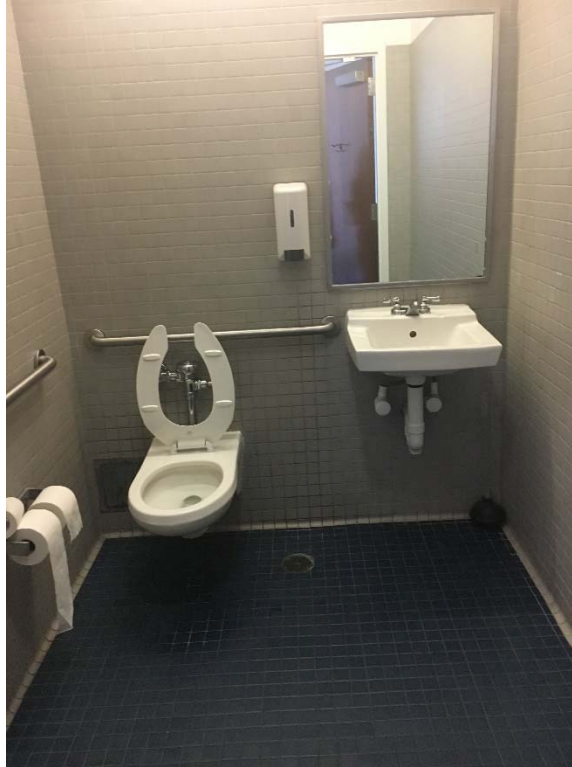
Violation 26 - 2nd floor Men's and Women's restrooms by the track - The lavatories encroach on the required clear floor width of the water closets.
