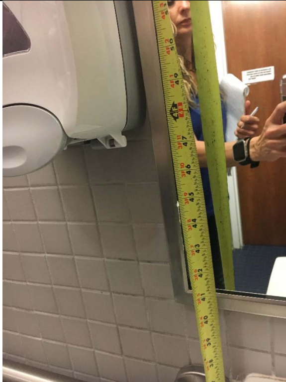
Violation 27 - 2nd floor Men's and Women's restrooms by track - The mirrors are mounted with the bottom of the reflective surface at 41" where a maximum of 40" is required.
