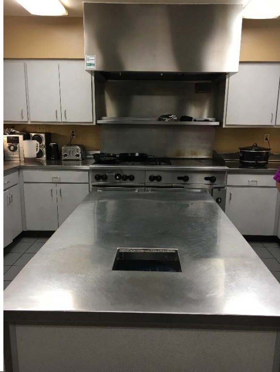
Violation 32 - The kitchen does not have a lowered section or workspace provided.
