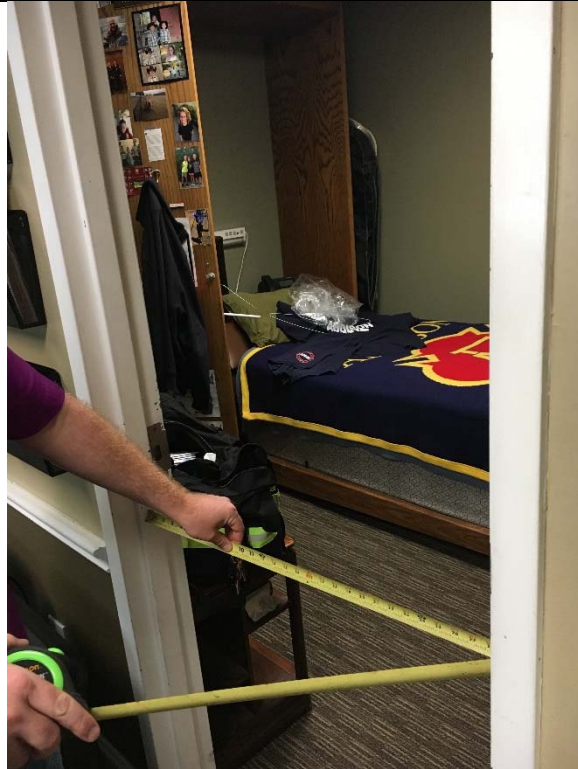
Violation 21 - Single sleep room door opening is only 29" wide where a minimum of 32" is required.
