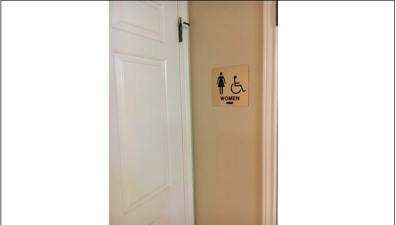
Violation 10 - Women's Restroom: Signage is mounted on the wall next to the hinge side of the door.
