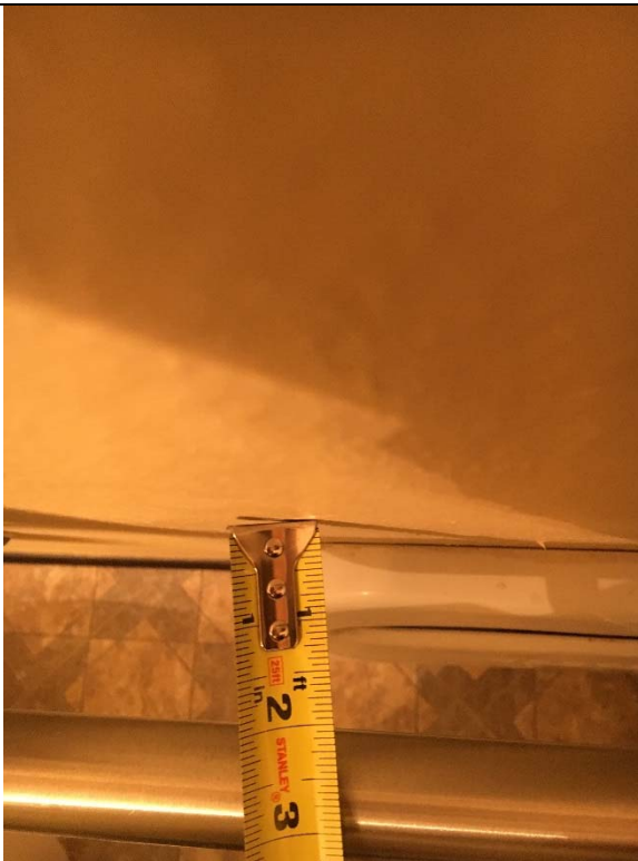
Violation 13 - Women's & Men's Restrooms: The space between the grab bar and the wall is 2".
