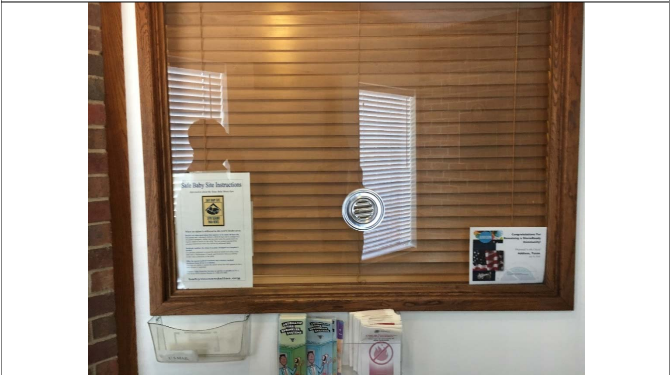
Violation 6 - The no-draft speak-thru at the entrance is at 52".
