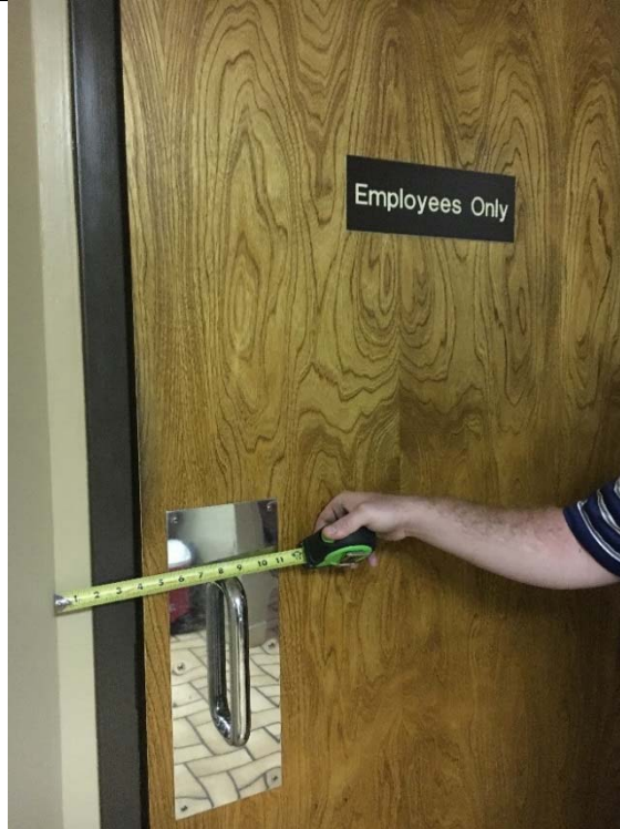
Violation 13 - The door into the Employees Only area only has a 4" maneuvering clearance on the pull side.
