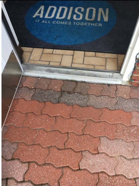
Violation 3 - The threshold at the exterior door leading into the vestibule has a threshold that is greater than 1/2".
