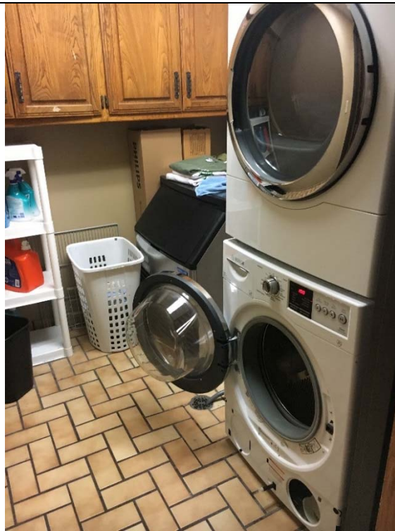
Violation 14 - The door leading into the laundry room only has a 4-1/2" maneuvering clearance on the pull side.
