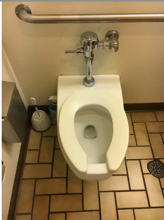
Violation 22 - The flush control in the Men's and Women's restrooms are mounted on the closed side.
