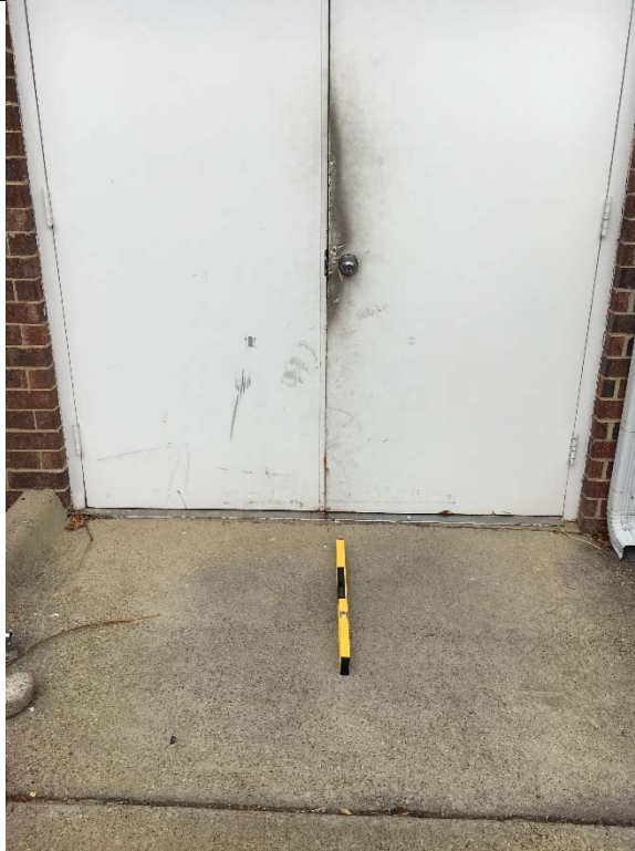
Violation 11 - The landing in front of the door leading into the weight room has a 6% slope.
