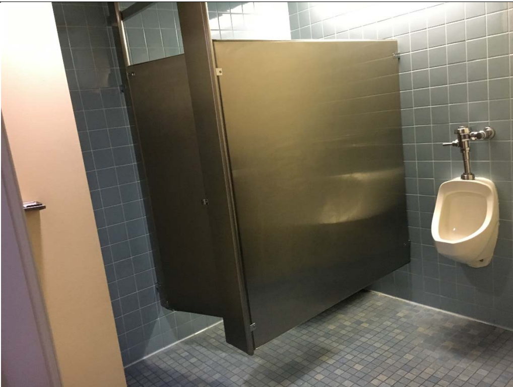
Violation 47 - Men's restroom on second floor - Door opening is only 30" where a minimum of 32" is required.
