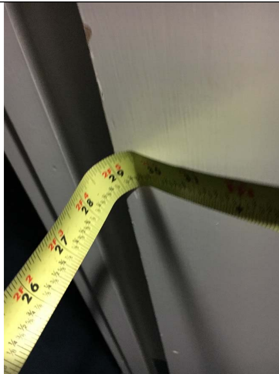
Violation 21 - The staircase in the main lobby hallway is at 62.5" with no protection.
