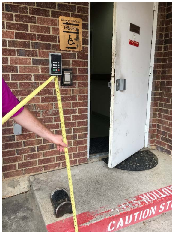
Violation 11 - The landing in front of the door leading into the weight room has a 6% slope.
