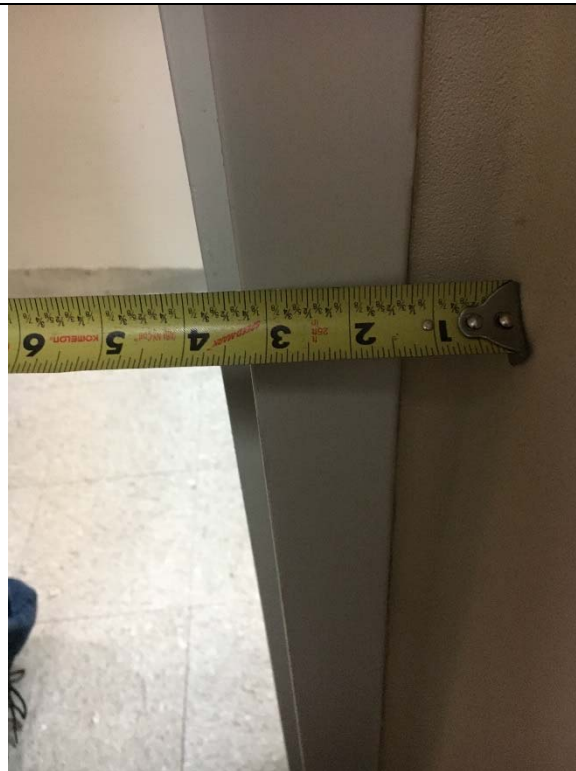
Violation 35 - There is only a 3-1/2" maneuvering clearance on the pull side as you exit the Women's locker room; a minimum of 18" is required.
