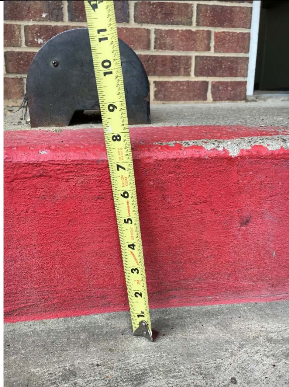
Violation 12 - The back entrance door for "Authorized Personnel Only" requires a 7.5" step up.
