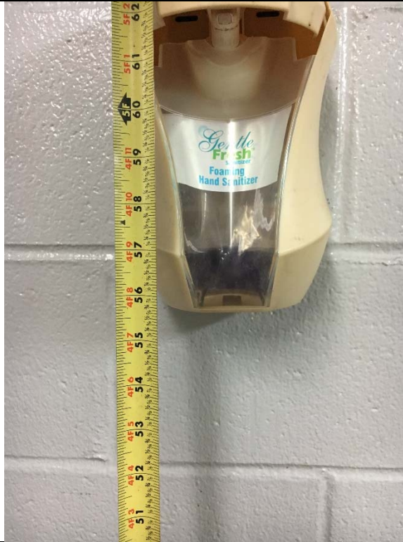
Violation 60 - Hand sanitizer dispenser in the gun range is mounted above the required 48".
