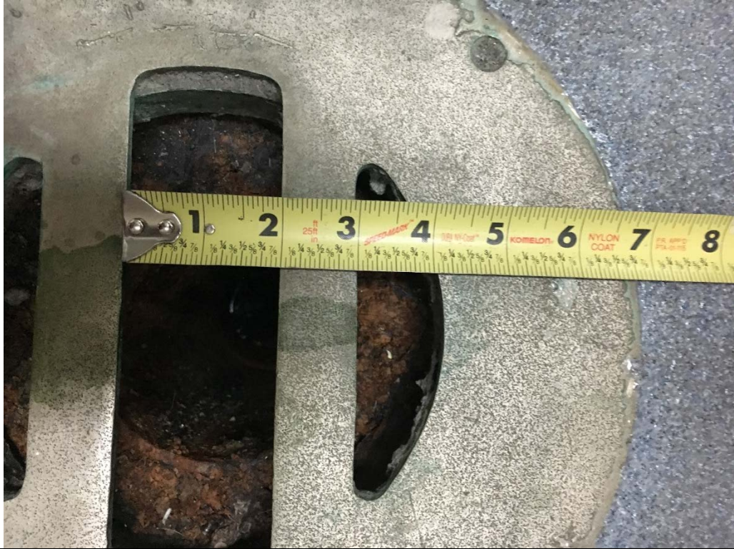
Violation 55 - There is a drain in the jail area with openings from 1"-2" wide.
