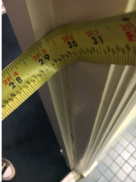
Violation 47 - Men's restroom on second floor - Door opening is only 30" where a minimum of 32" is required.
