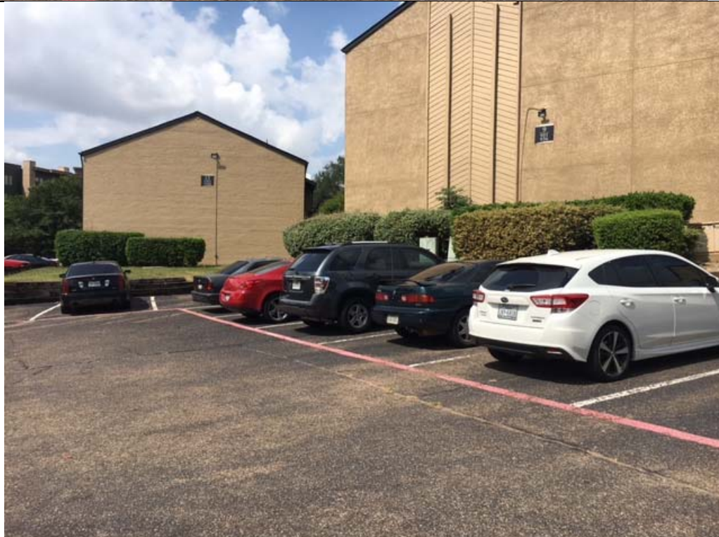
Violation 1 - There are no accessible parking spaces provided to serve this parking lot.
