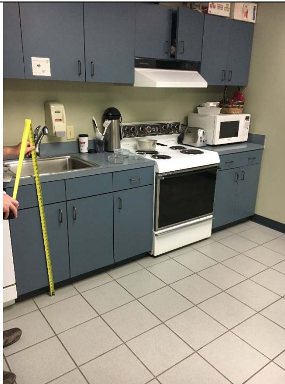
Violation 44 - The counter/sink in the 1st floor break room is at 36 5/16" above finished floor.
