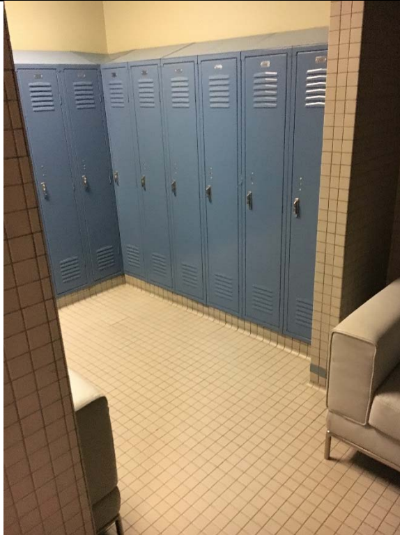
Violation 27 - Breakroom Area: Women's room locker area does not have an accessible bench.
