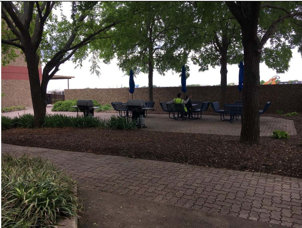
Violation 52 - The outdoor seating area does not have any accessible picnic tables provided.
