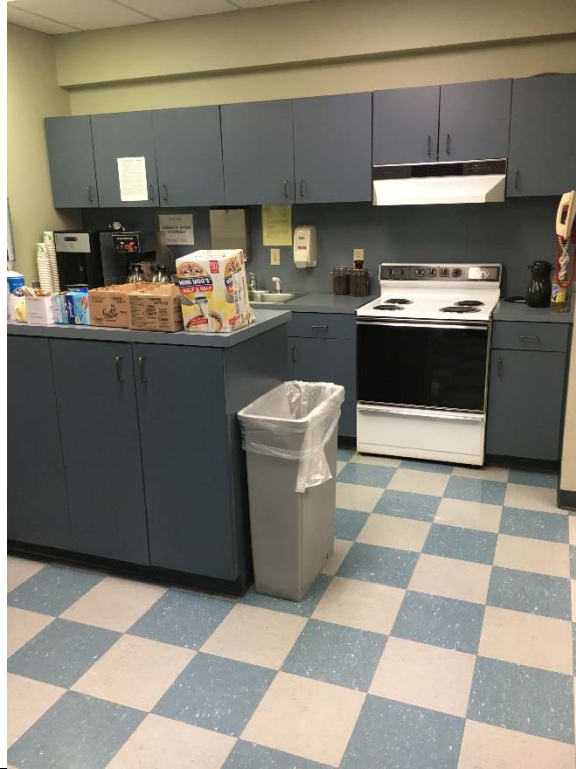
Violation 44 - The counter/sink in the 1st floor break room is at 36 5/16" above finished floor.
