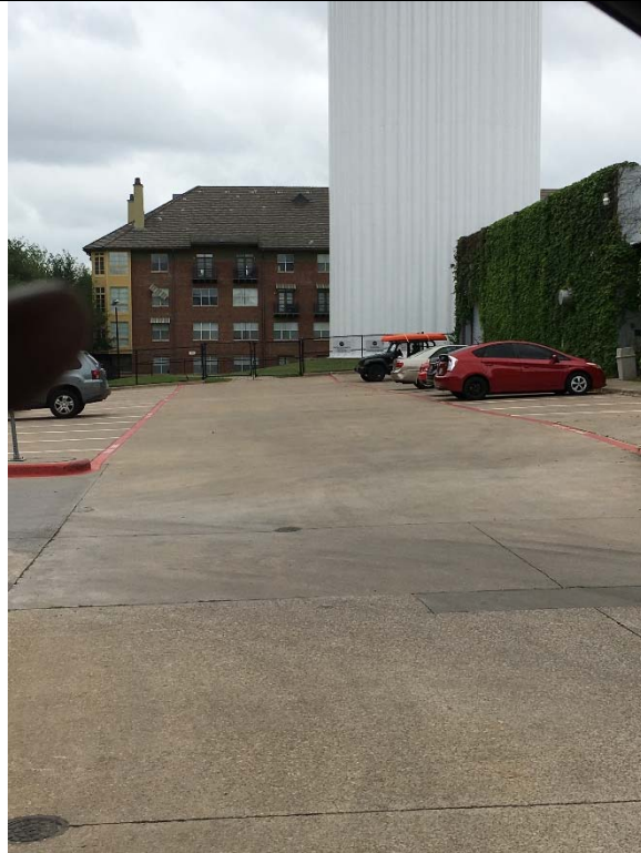
Violation 1 - There are no accessible parking spaces provided in the employee parking lot.
