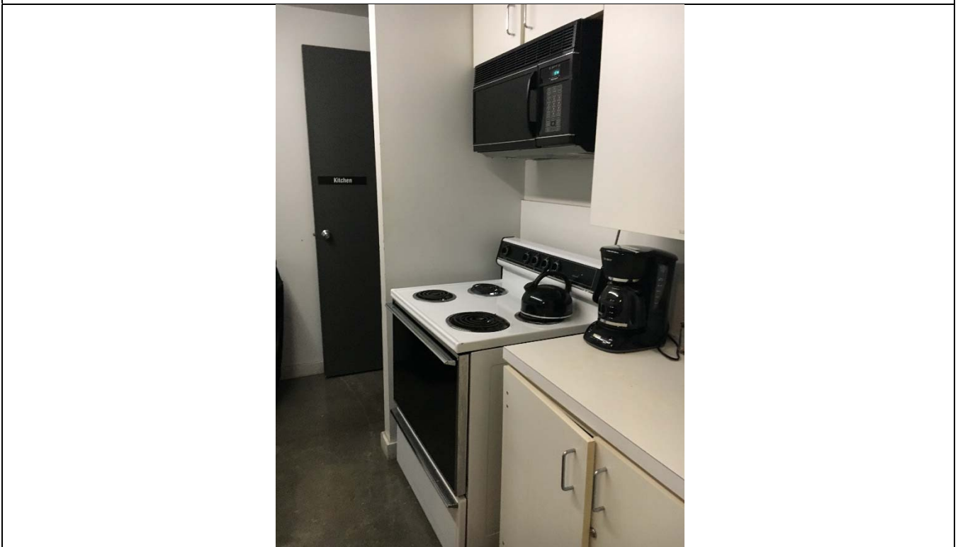
Violation 16 - The microwave provided is mounted above the stove and out of reach.
