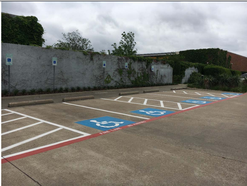
Violation 2 - Two of the accessible parking spaces are not a minimum of 96" wide: The third space is 92-1/2" wide and the fifth space is 93" wide.
