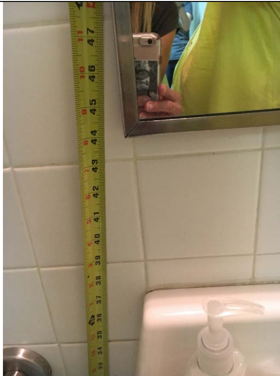
Violation 39 - Men's Room: Mirror is at 44-1/2" to the bottom of the reflective surface.
