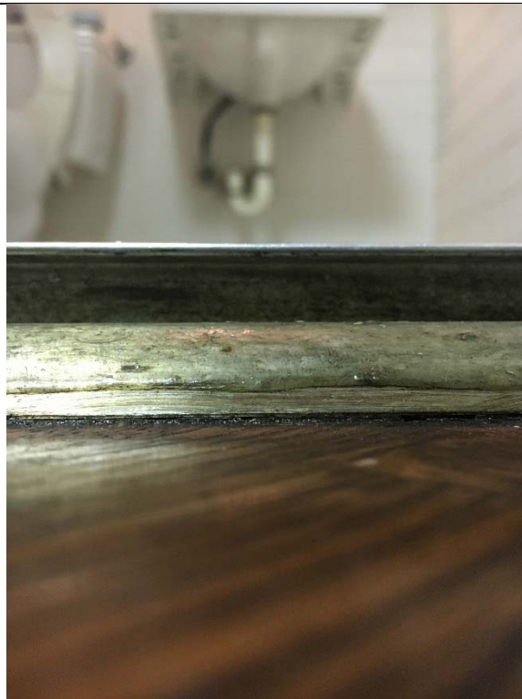
Violation 35 - Men's Room: There is a 1-3/4" step to get into the restroom.
