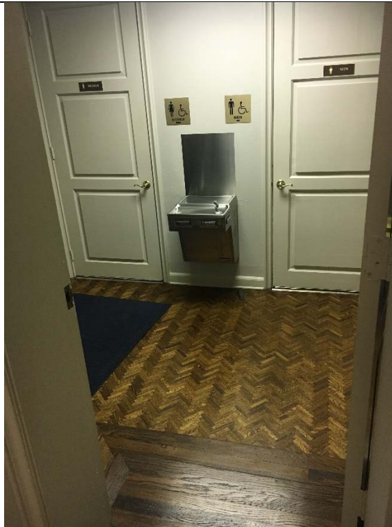
Violation 48 - There is only one drinking fountain provided, where two are required.
