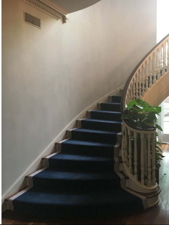
Violation 5 - There is no accessible route to the 2nd floor.
