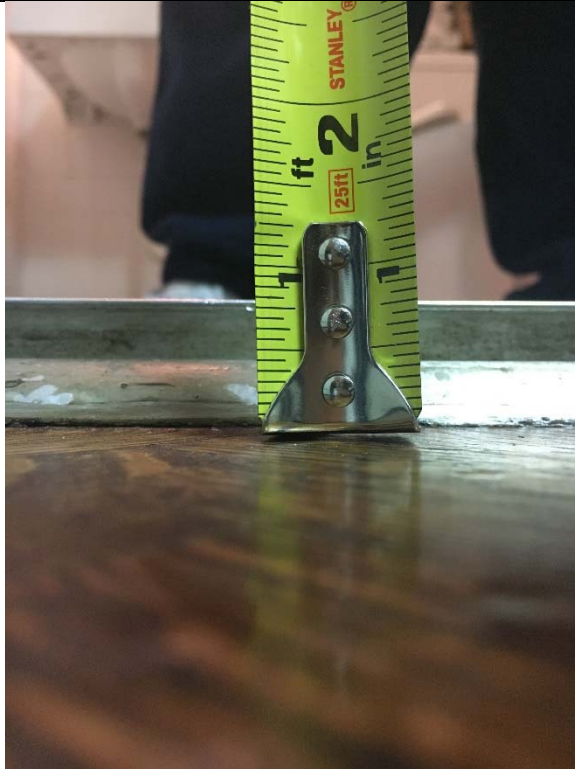
Violation 23 - Women's Room: There is a 1-3/4" step to get into the restroom.
