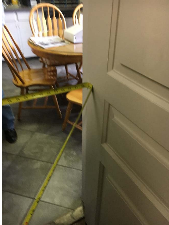
Violation 46 - The door width leading into the break room is only 29" wide.
