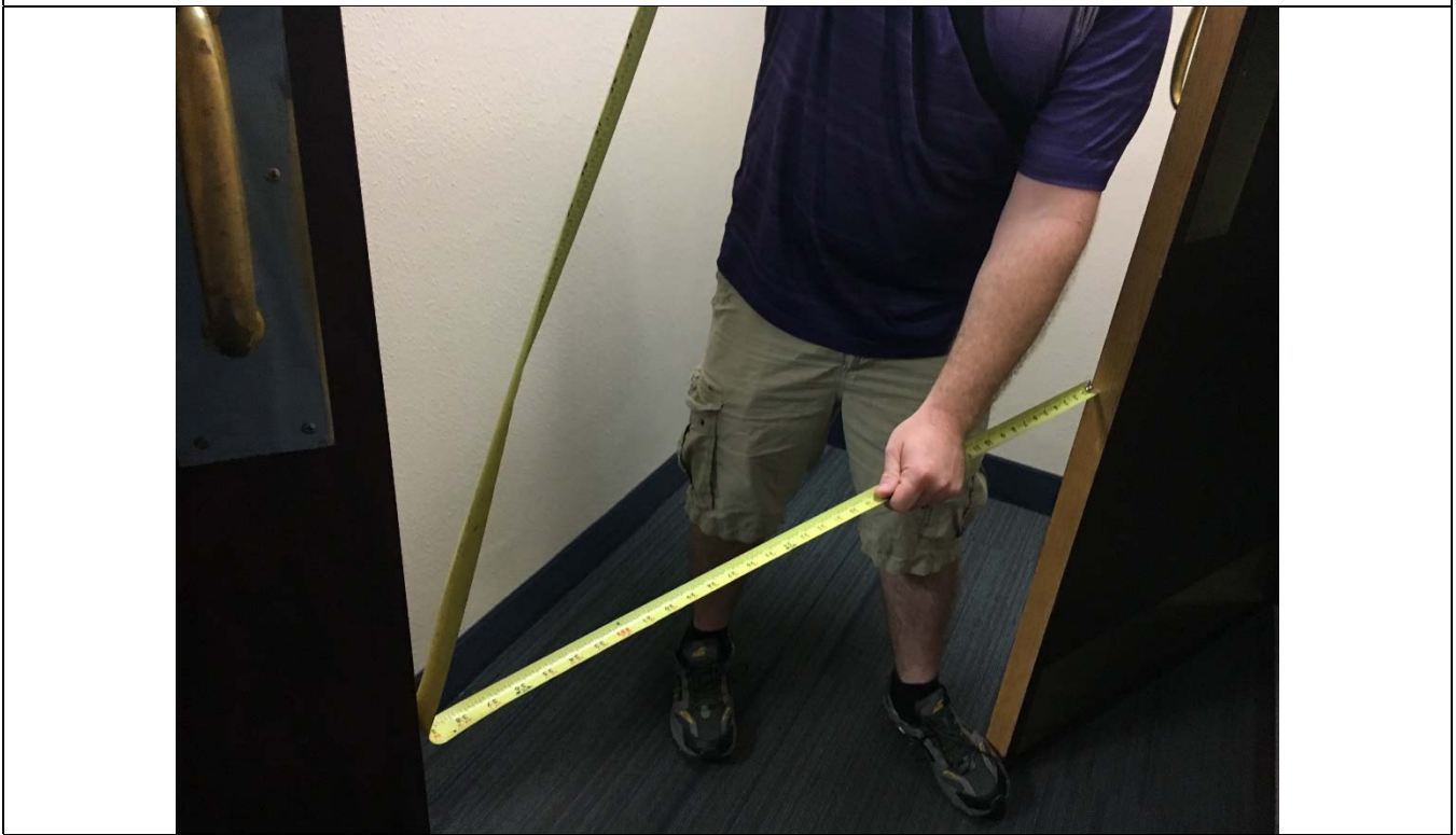
Violation 12 - The Women's restroom maneuvering clearance between two doors in a series is only 39" between doors.
