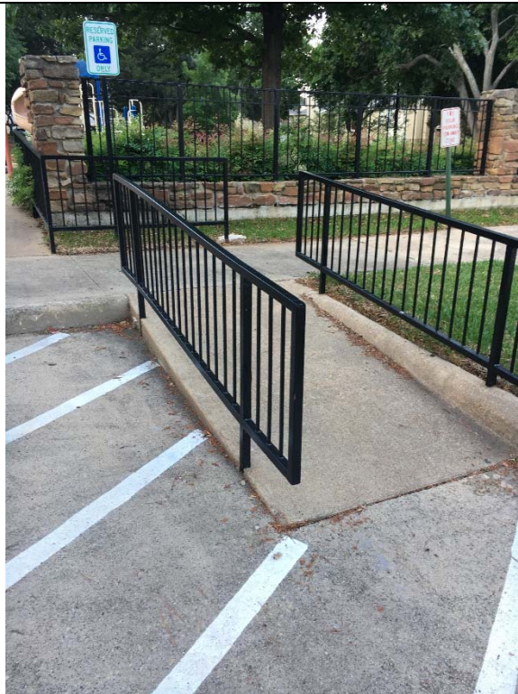
Violation 3 - The access aisle narrows down to 55" wide where the ramp is located.
