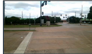
Corner 4 No Ramp (4z)
