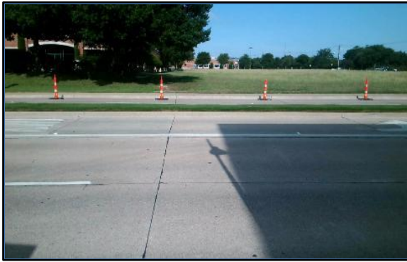
Corner 1 No Ramp (1z)
