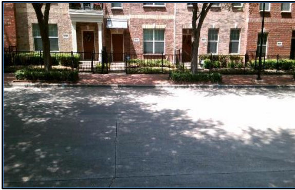
Corner 1 No Ramp (1z)
