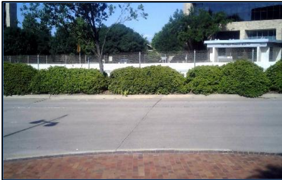
Corner 3 No Ramp (3z)
