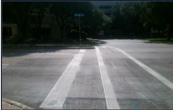
Corner 2 No Ramp (2z)
