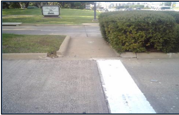
Ramp West F
