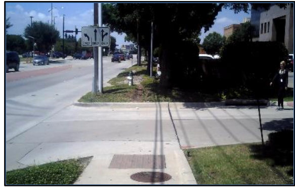
Corner 2 No Ramp (2z)
