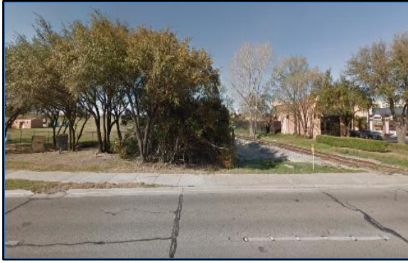
Corner 1 No Ramp (1z)
