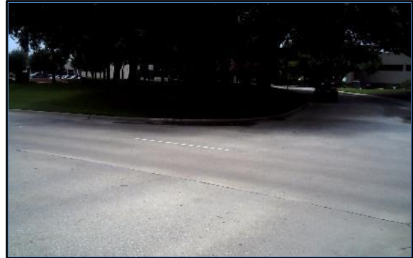
Corner 4 No Ramp (4z)
