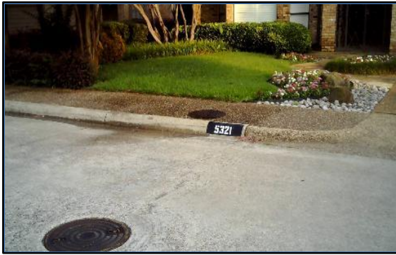
Corner 1 No Ramp (1z)
