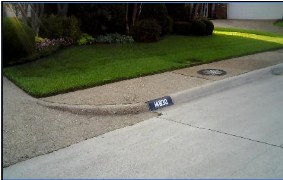
Corner 3 No Ramp (3z)
