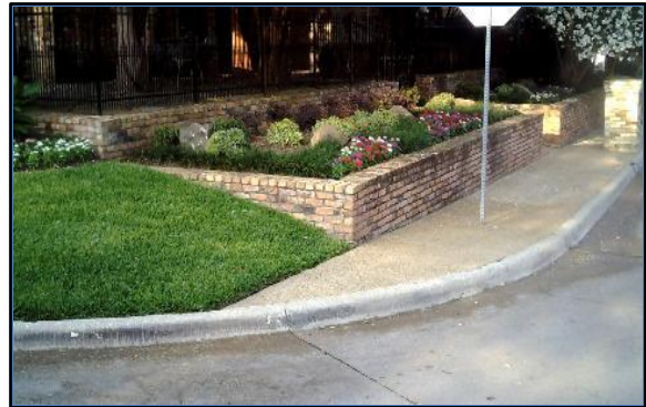
Corner 4 No Ramp (4z)
