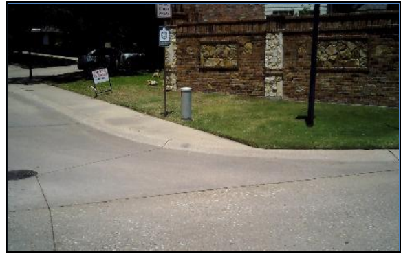
Corner 2 No Ramp (2z)
