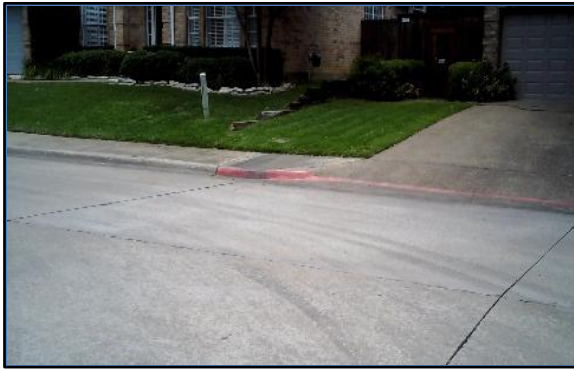
Corner 2 No Ramp (2z)
