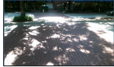
Ramp South F
