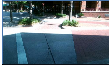
Ramp East F
