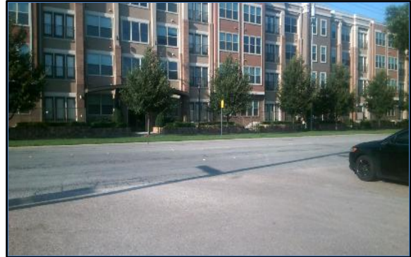
Corner 4 No Ramp (4z)
