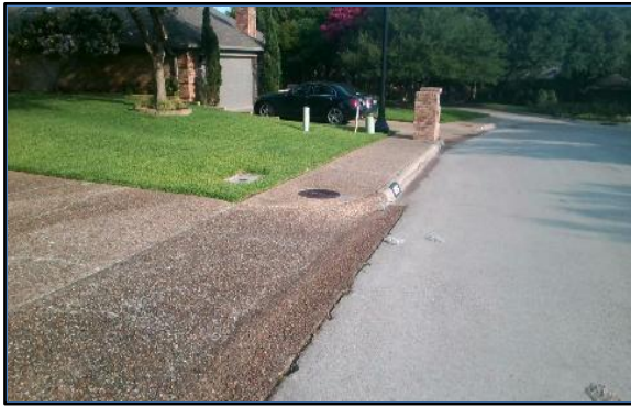
Corner 1 No Ramp (1z)
