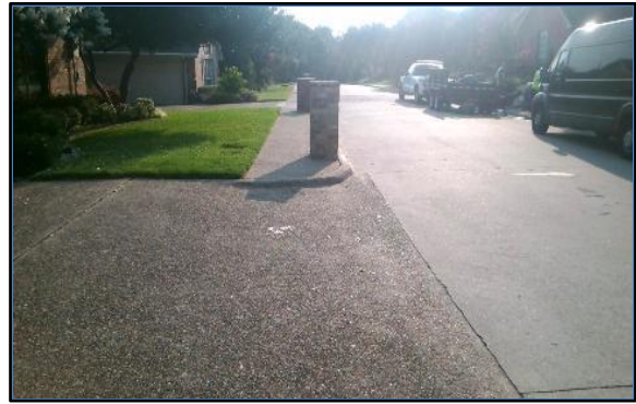
Corner 2 No Ramp (2z)
