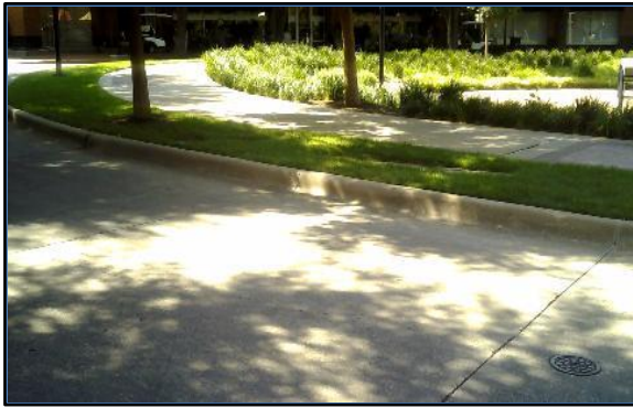
Corner 1 No Ramp (1z)
