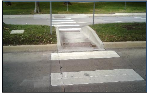
Ramp North G
