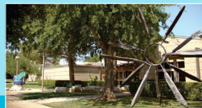
Fine and Performing Arts Center, 1973 Architects: Pratt, Box, Henderson and Partners Renovation: Hidell and Associates, 1995
