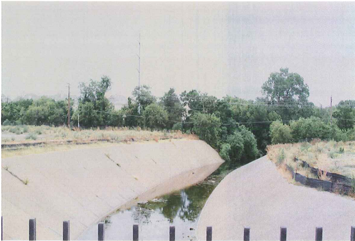
UPSTREAM VIEW FROM BRIDGE LOOKING EAST
