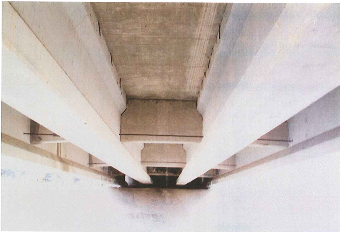
SUPERSTRUCTURE LOOKING SOUTH
