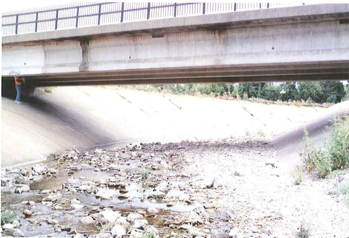
STREAM VIEW LOOKING EAST
