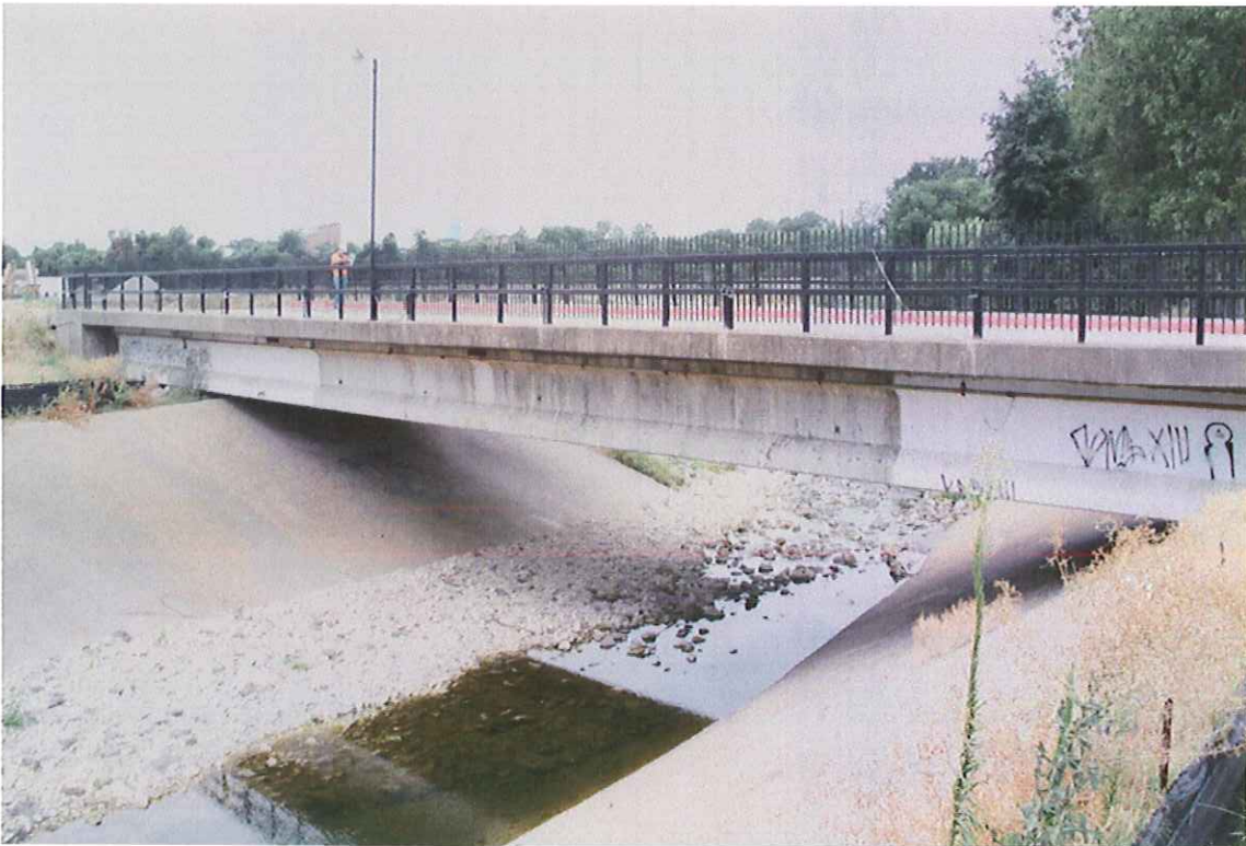
BRIDGE ELEVATION LOOKING EAST
