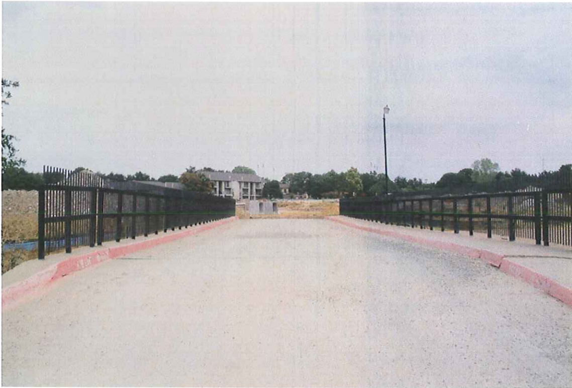
BRIDGE ROADWAY LOOKING NORTH
