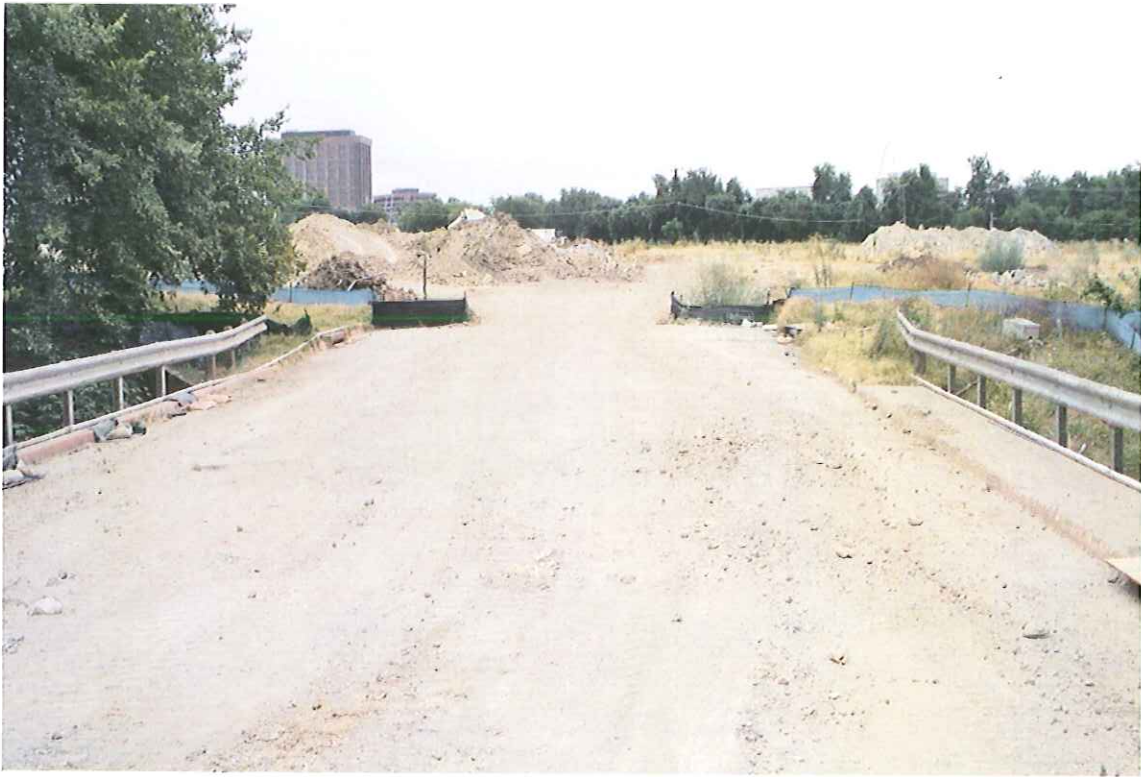
BRIDGE ROADWAY LOOKING EAST
