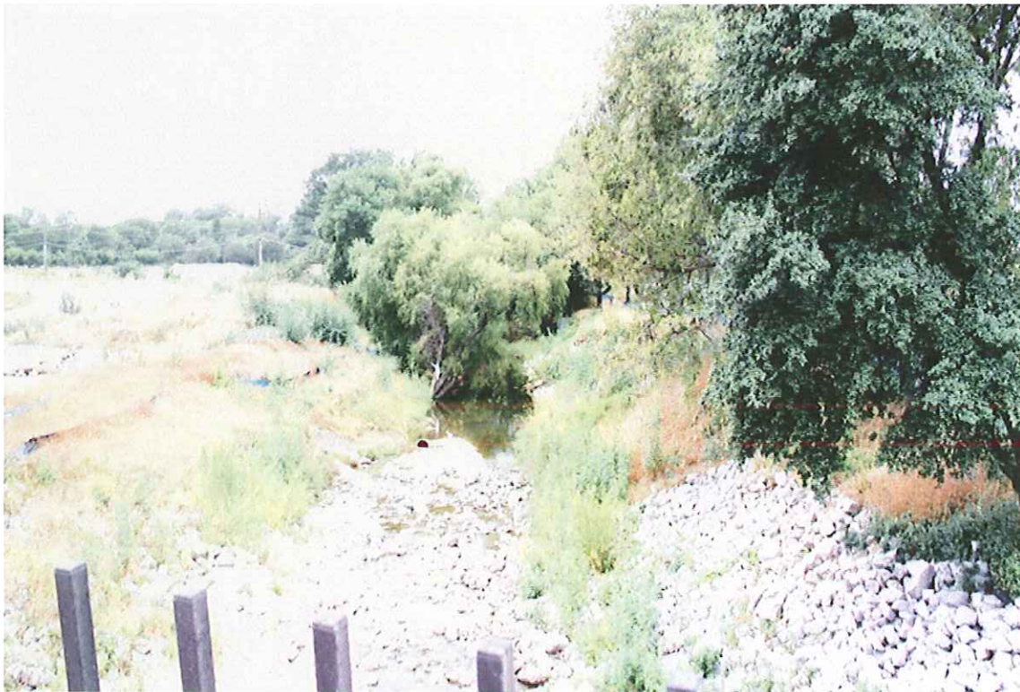
DOWNSTREAM VIEW FROM BRIDGE LOOKING WEST
