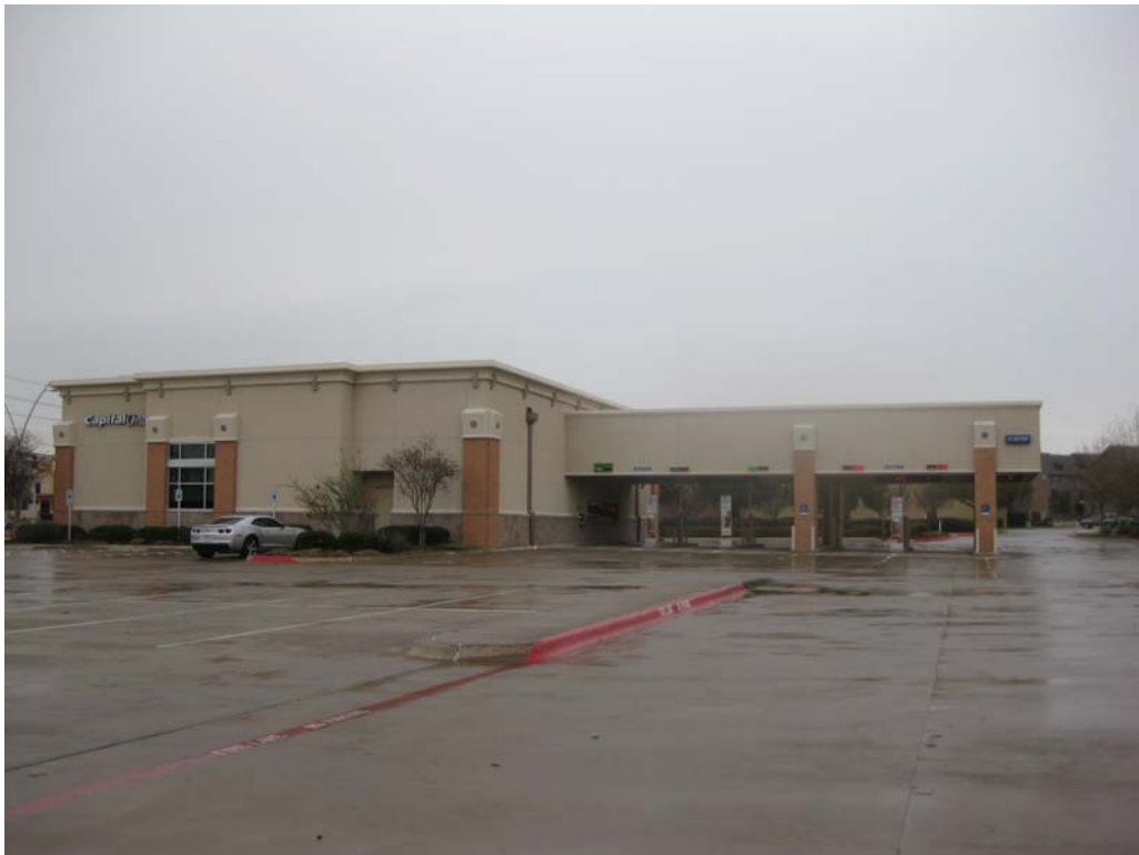
Subject Building and Drive-Through Canopy
