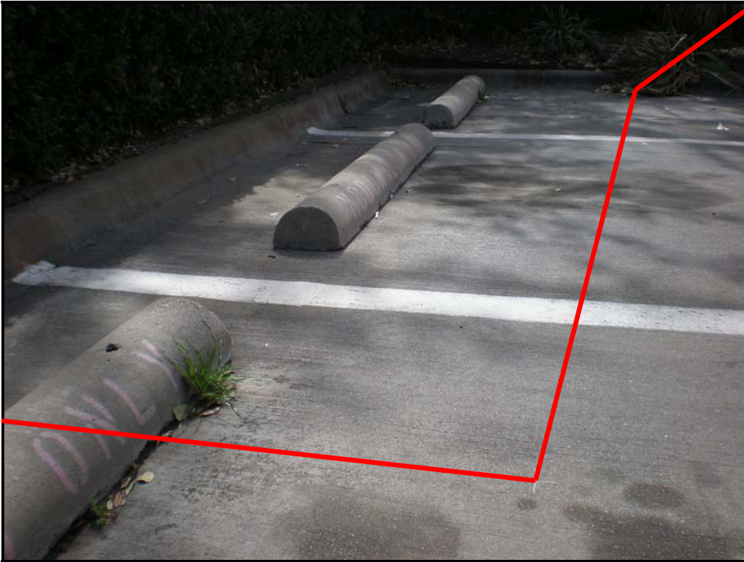
Looking south at the parking spaces affected by the proposed permanent easement, with the estimated boundary in red, x-cut found on pavement.
