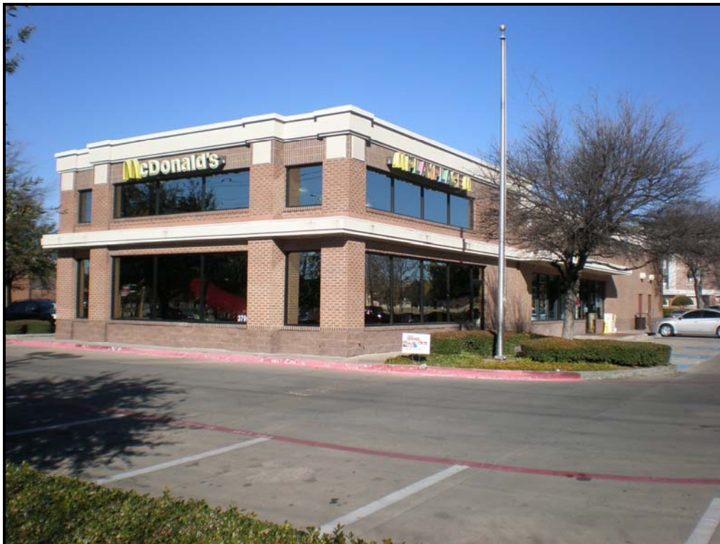
Looking north at the restaurant building.
