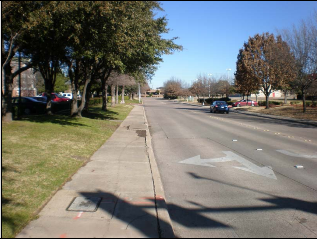
Looking north along Business Avenue, subject at left.
