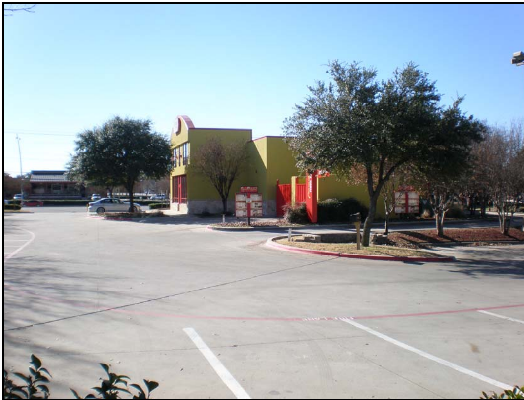
Looking south at the rear of the subject.
