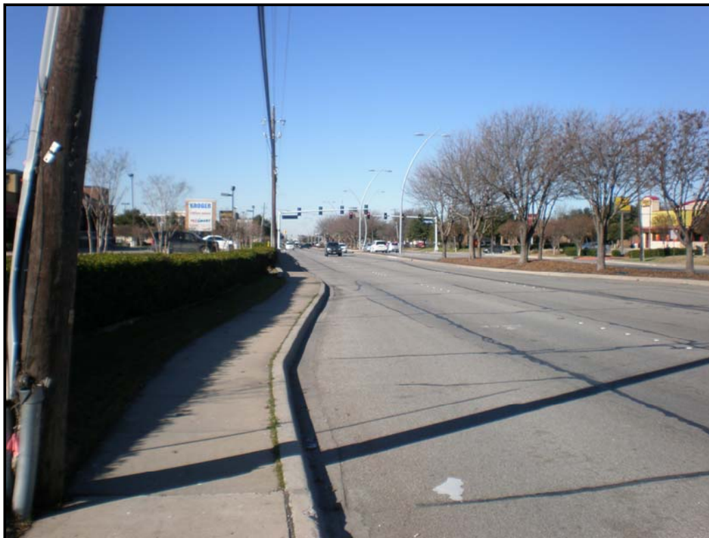
Looking west along Belt Line Road, subject at left.
