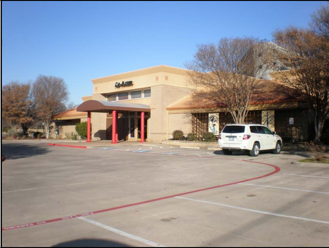
Looking north at the restaurant, not affected or appraised herein.
