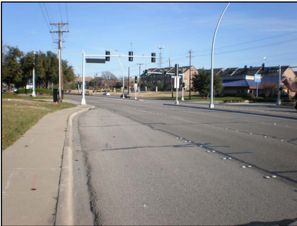
Looking east along Belt Line Road, subject at left.
