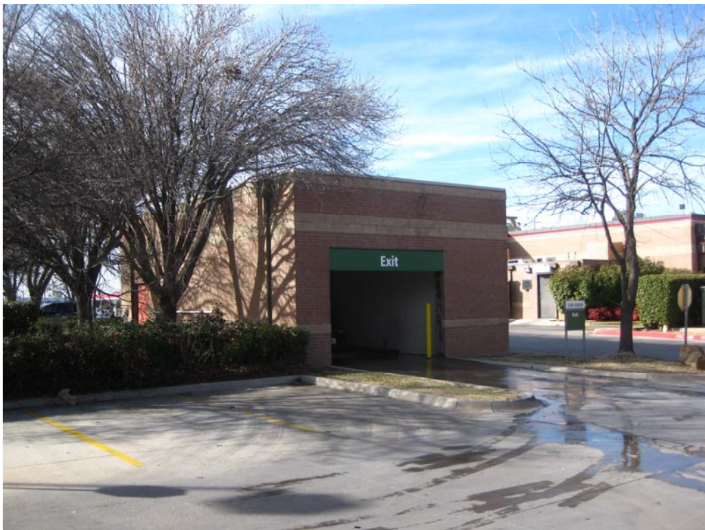
Car Wash Facility
