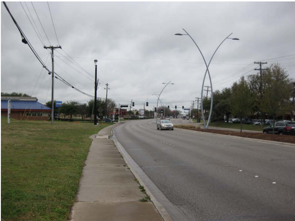
Belt Line Road, Looking West; Subject on Left.
