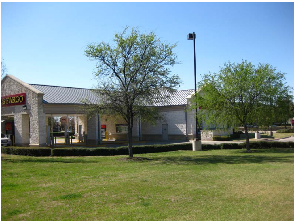
Drive Through Canopy
