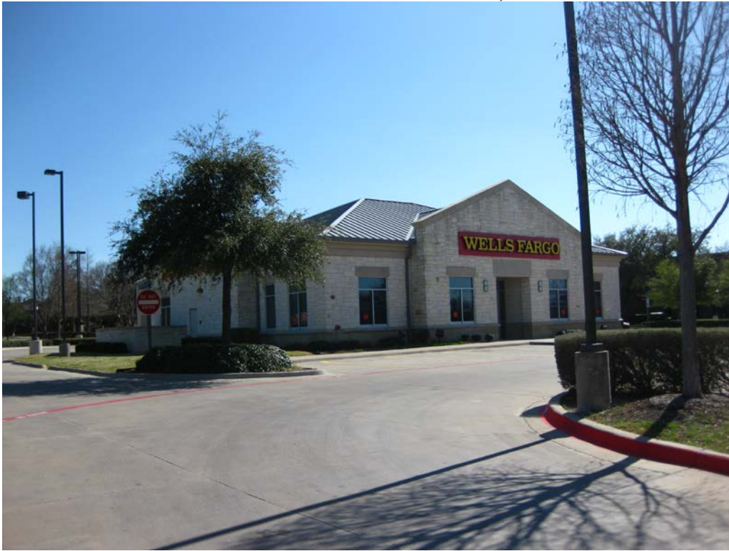
North Side of Building, Facing Belt Line Road
